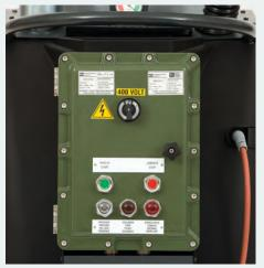
Motor and electrical parts are IECEx marked
